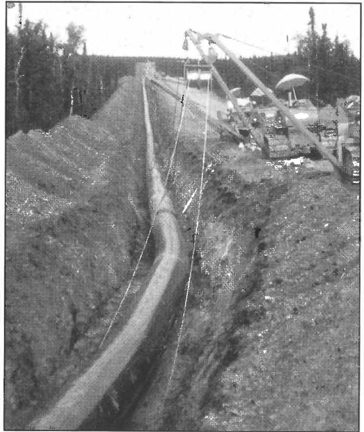
Plattline™ installation on 387 miles of the Aleskya Pipeline.
